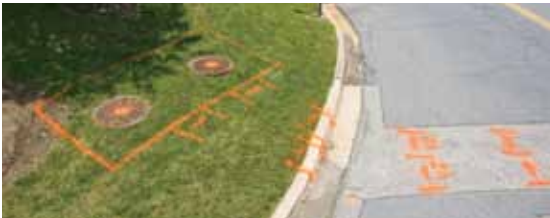
Example of conduits, underground structure
