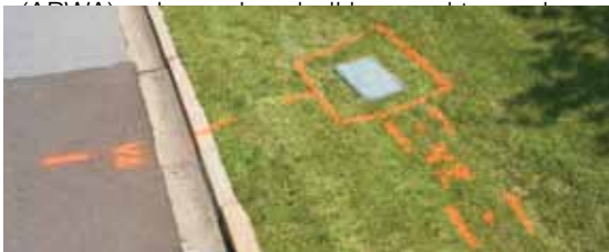
Example of structure, standard marks, corridor
